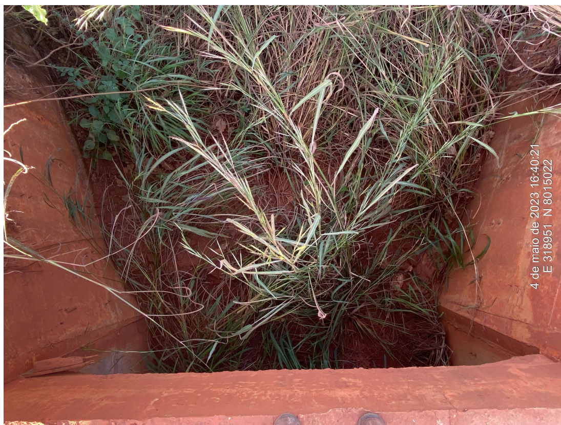
Km 19,10 – Bueiro Celular existente BSCC 2,0x2,0
