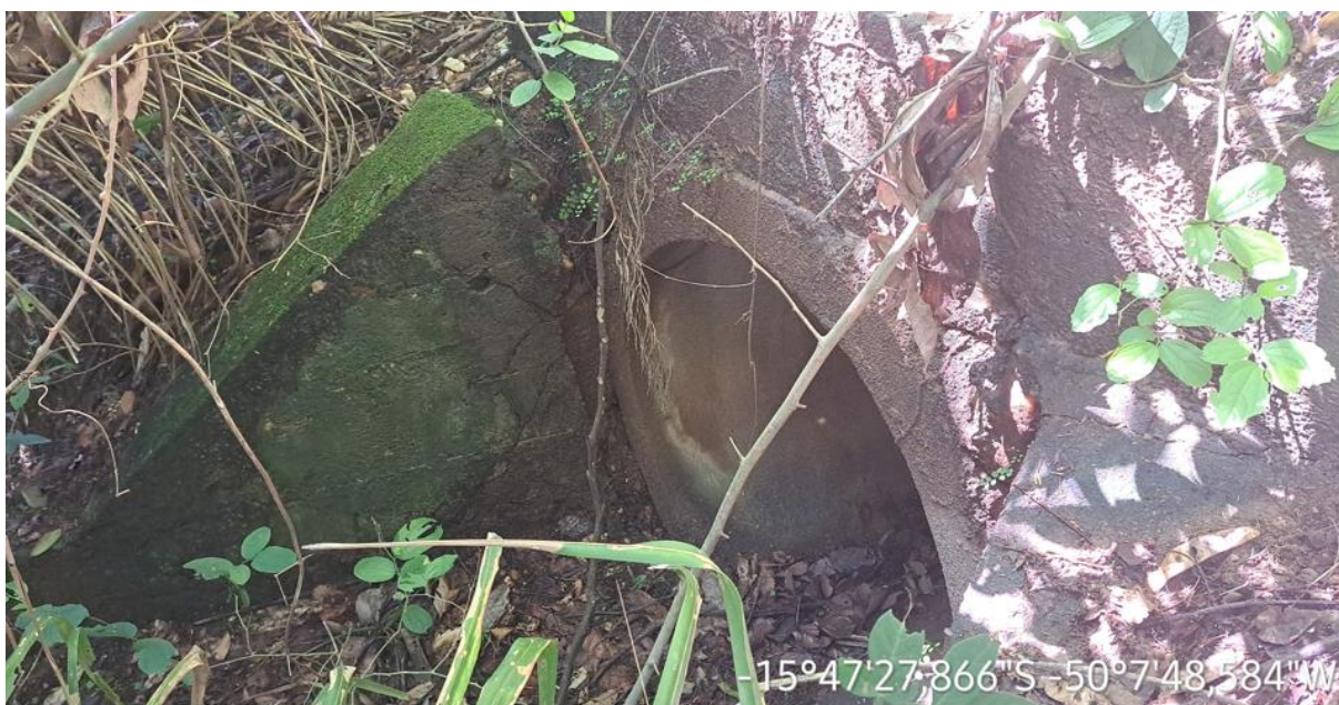
-15°47'27.866"S -50°7'48.584"W Km: 21,00 – Bueiro tubular.
