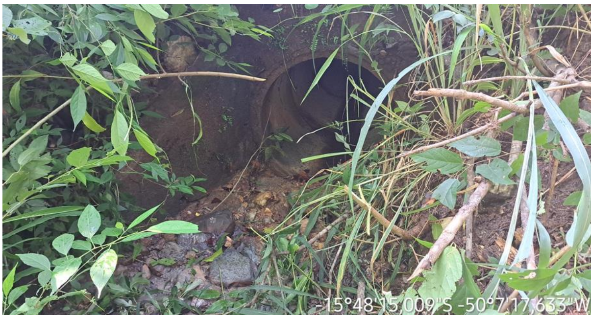
-15°48'15.009"S -50°7'17.633"W Km: 19,30 – Bueiro tubular.
