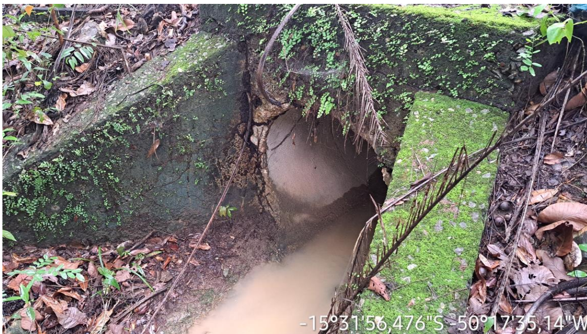
-15°31'56,476"S -50°17'35,14"W Km: 55,70 – Bueiro tubular.
