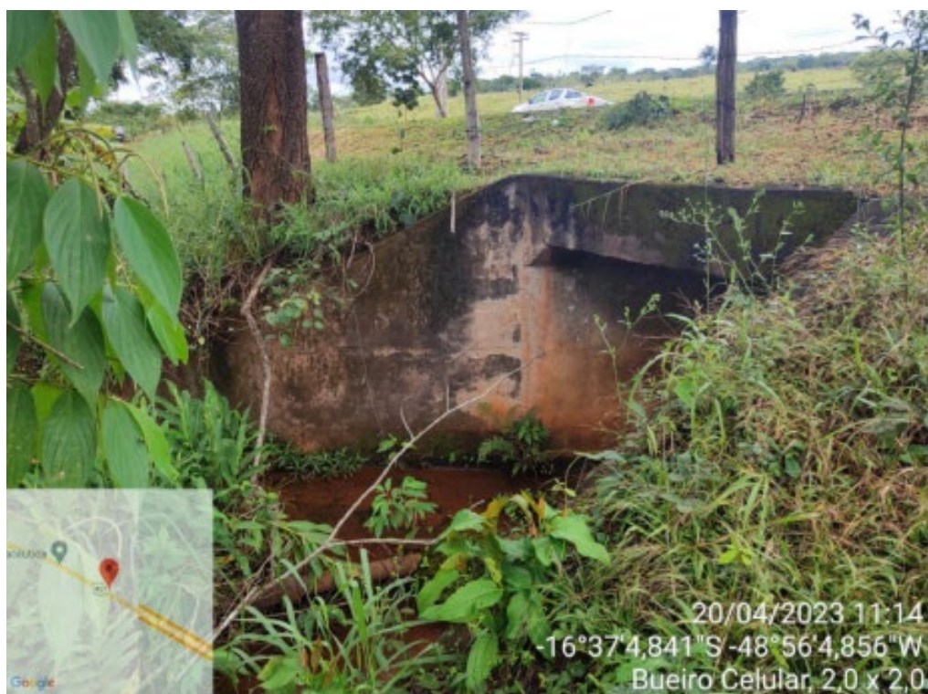
Km 16,6 – Bueiro existente BSCC 2,0x2,0.
