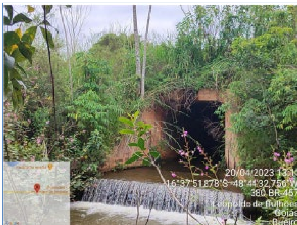
Km 38, 1 O - Bueiro existente BSCC 2,0x2,0.
